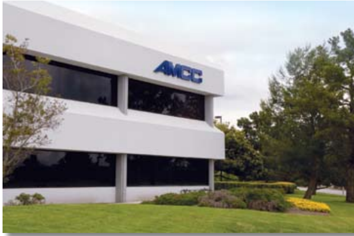
AMCC Headquarters in Sunnyvale, CA
